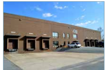
Conover, North Carolina Dispenser Manufacturing
